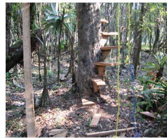
A new tree based bird-watching tower under construction
