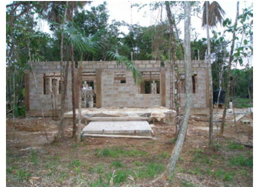
Hummingbird Model Home Under Construction
