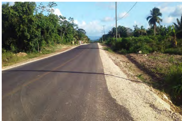
Newly Paved Frank Eddy Main Road
